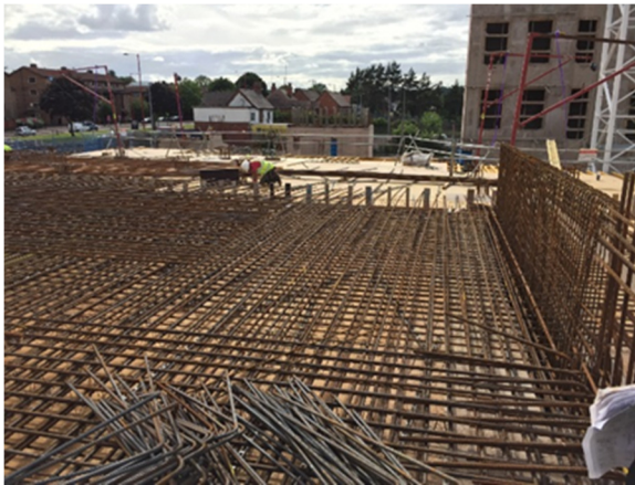
Steel fixing at the 450mm thick transfer slab
