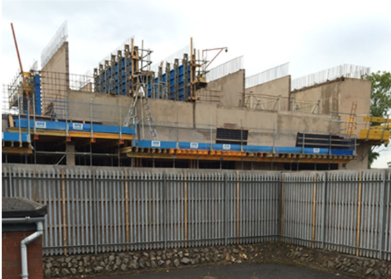
Cross walls under construction at Level 1
