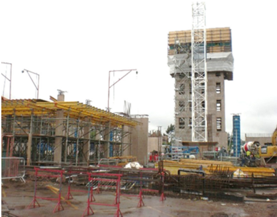
The slip-formed central lift and stair core
