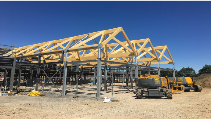
Erection of Dining Hall Roof
