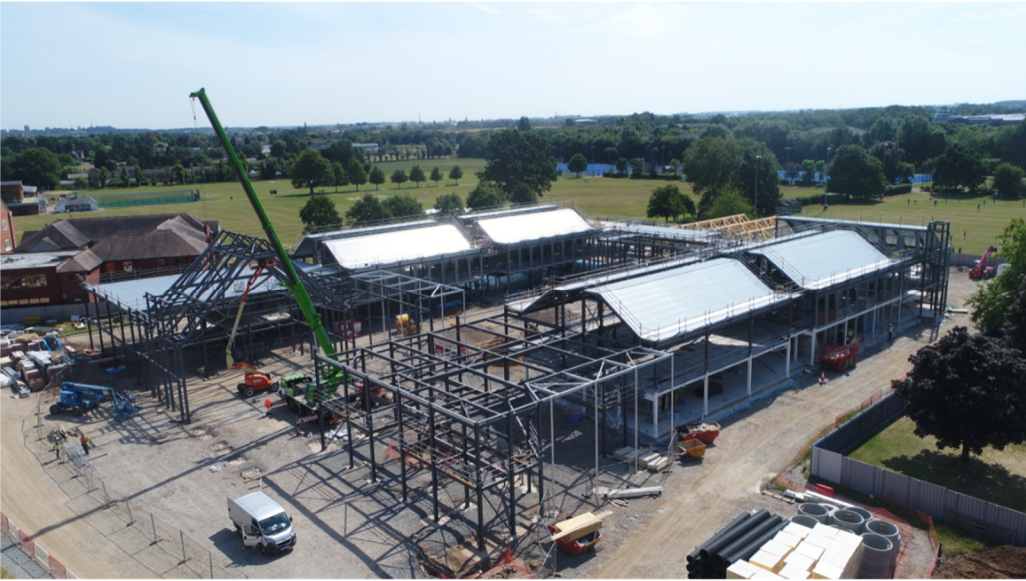
Erection of steel frame
