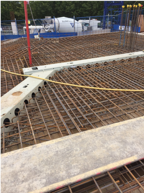
Delta Transfer Beams during construction prior to casting concrete
